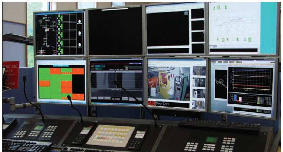
A view of the control screens. The TIM Video Viewer is in the bottom row, third from left.
