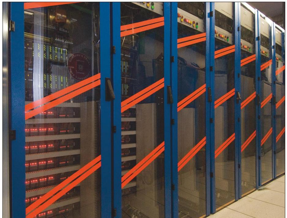
*The Detector Safety System used in the LHC experiments is one of many control systems.*
